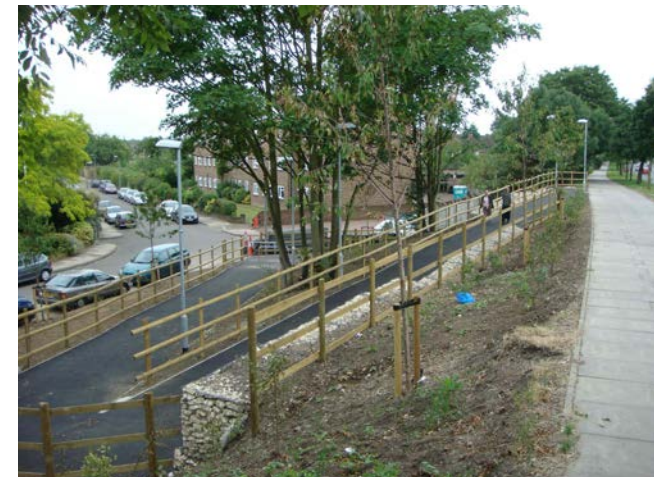
Access ramp, Richmond
