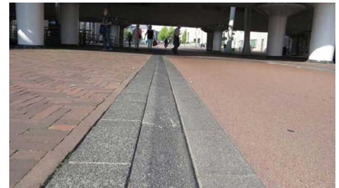
Angled kerbs as used in London, above and the Netherlands, below. Note that block paving should only be used over short distances, if at all, because it can be uncomfortable to ride over
