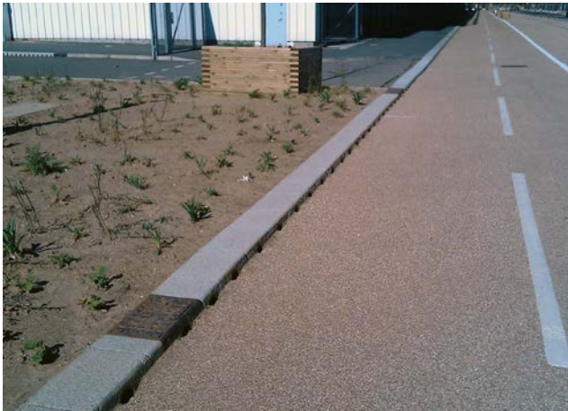
Perforated kerb gullies, as used in a cycle track
