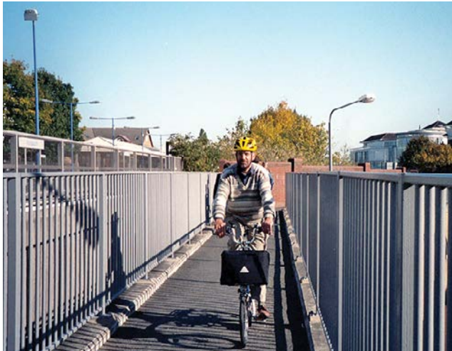
High bridge parapets
